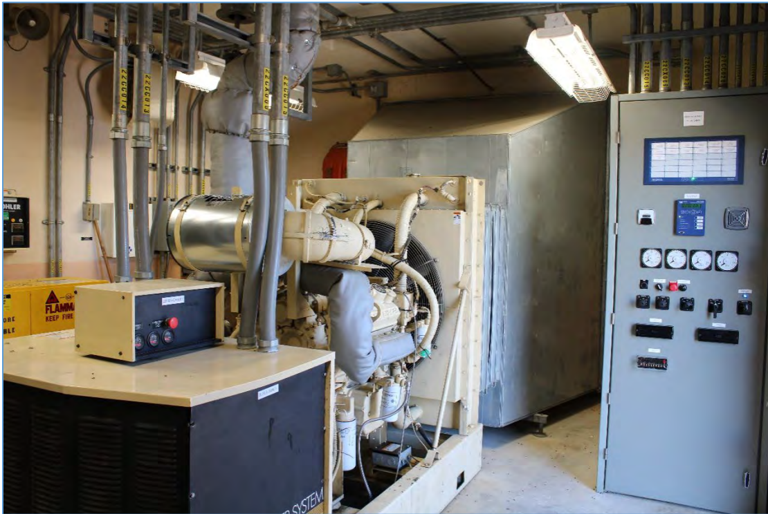
Figure 51: Diesel powered back-up generator in control building of Main Dam.
