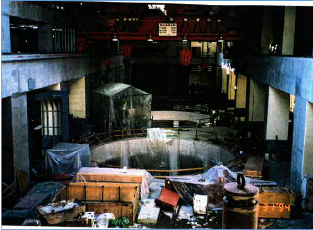
Figure 19: Construction progress of the Powerhouse Generator Bay from the erection bay (Source: OPC 1994).
