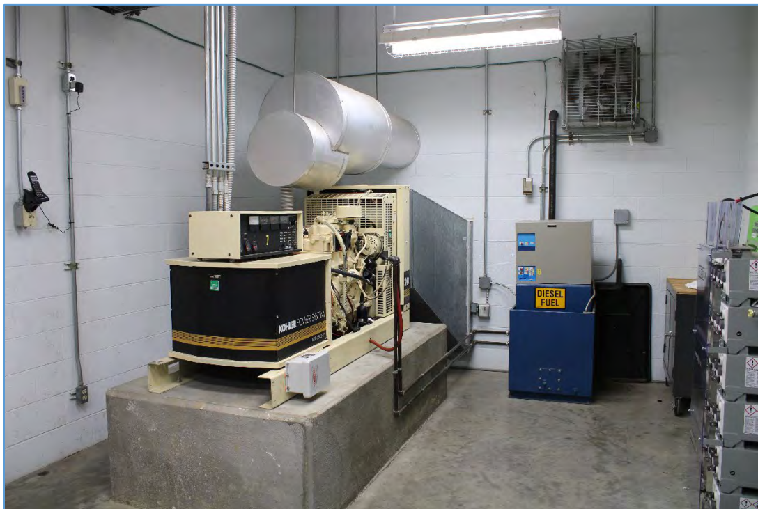
Figure 77: Back-up diesel generator located in communications buildings.
