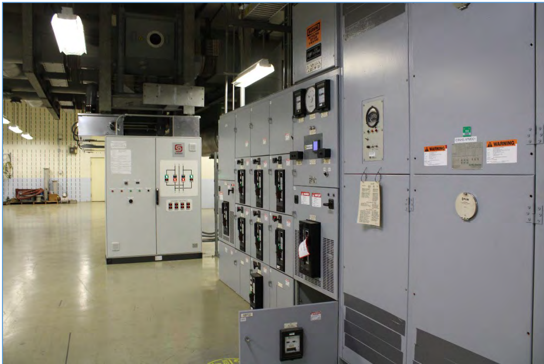
Figure 32: In-house substation that provides power to generators.
