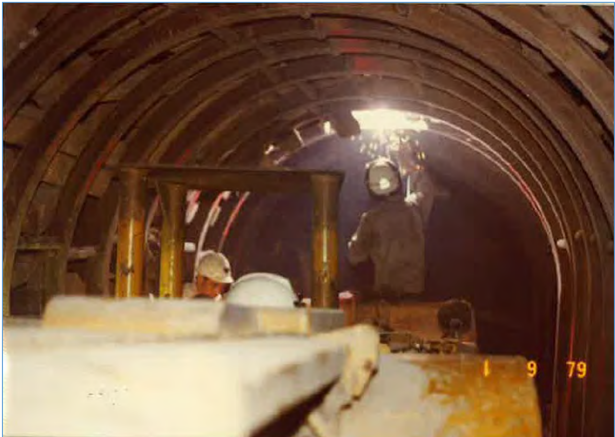
Figure 11: Workers shoring material supporting side walls of Powerhouse tunnel (Source: GPC 1979).
