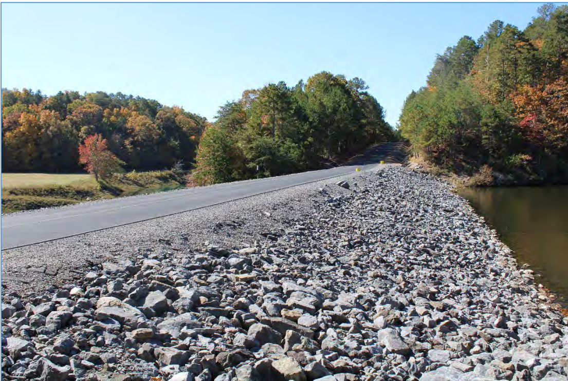
Figure 62: Rockfill on northwest elevation of Dam F adjacent to Auxiliary Pool I West, looking south.
