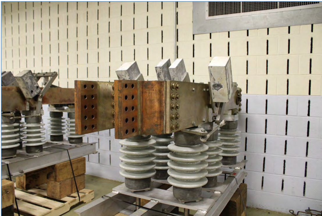
Figure 37: Old phase reversal switch.
