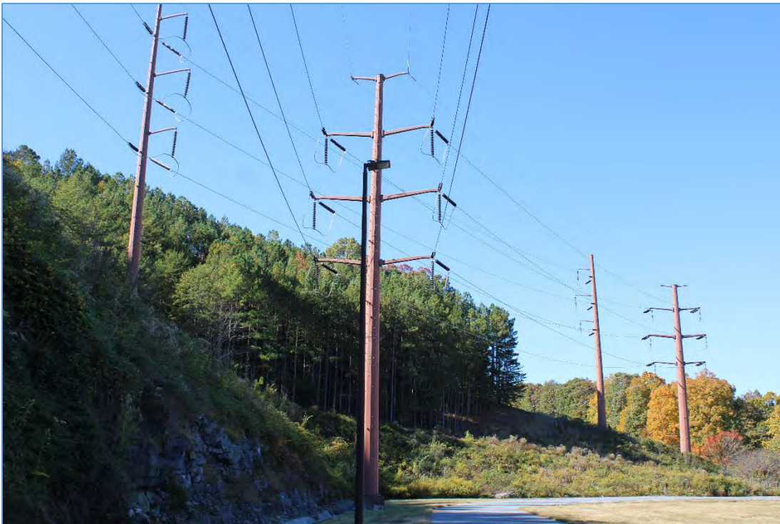
Figure 74: Primary Transmission line extending between the powerhouse transformers and substation, looking west.
