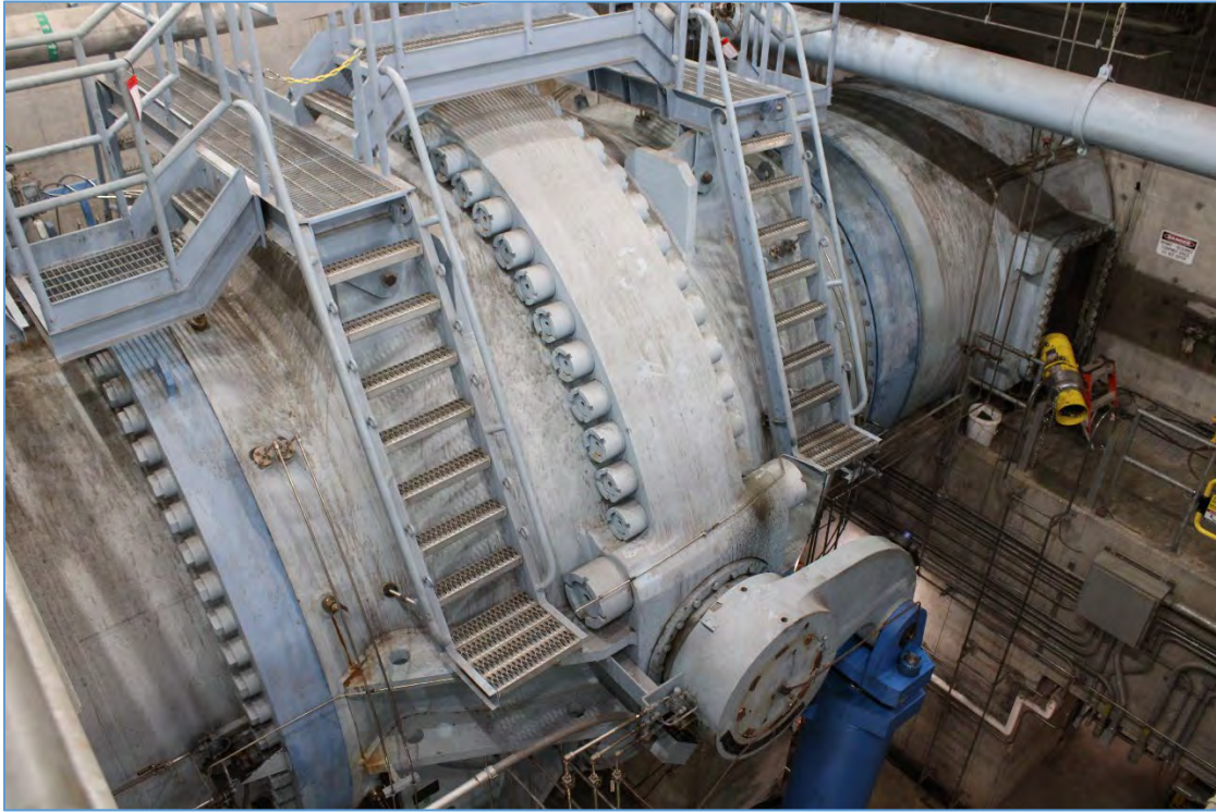
Figure 38: Inlet valve of Unit 3. Water flows through inlet valve before entering the turbine.
