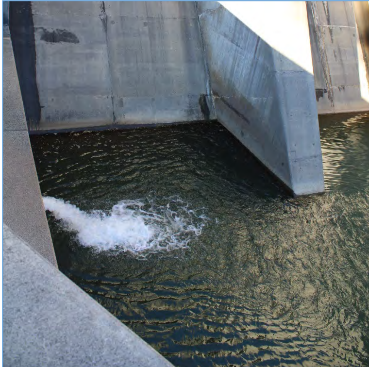
Figure 48: Minimum flow outlet at base of spillway at the Main Dam.
