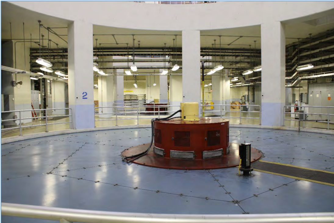
Figure 35: Top of Unit 2 and Unit 3 generator.
