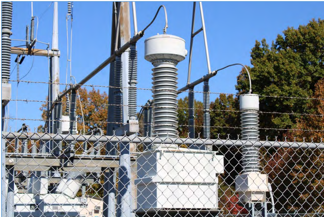
Figure 72: Lightning arrester in substation.
