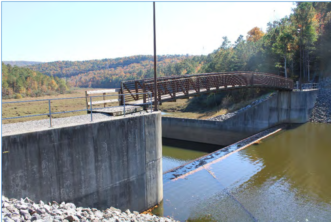
Figure 65: Formed concrete spillway at Auxiliary Pool II (Heath Lake), looking south.
