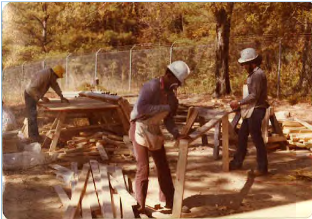
Figure 10: Photo of worker fabricating the construction office slab forms, taken October 18, 1978 (Source: GPC 1978).
