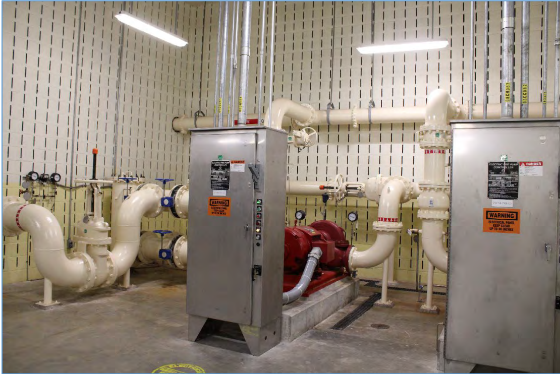
Figure 31: Primary and backup fire water system.
