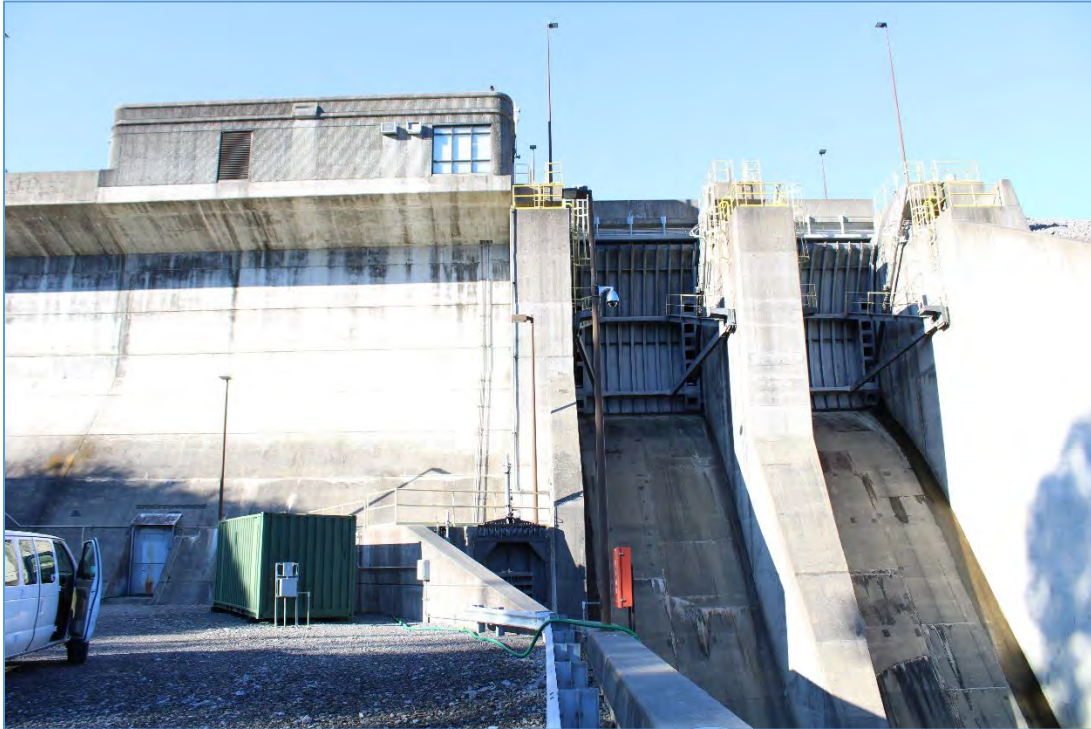
Figure 47: View of spillway and two Tainter gates and control building at Main Dam, looking west.
