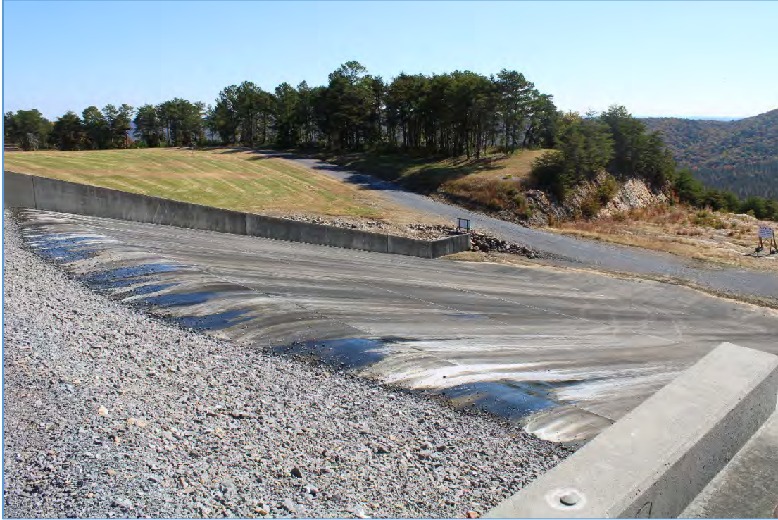
Figure 43: Gravel and formed concrete over-pump spillway, looking east.
