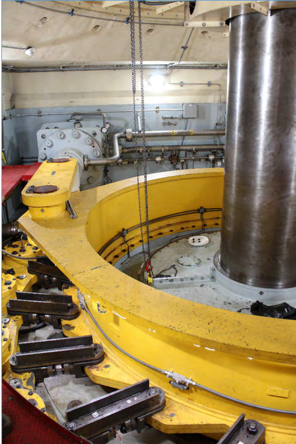
Figure 39: Turbine Pit Shaft.
