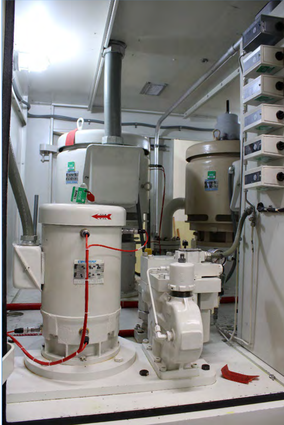
Figure 33: Governor Actuator Cabinet.
